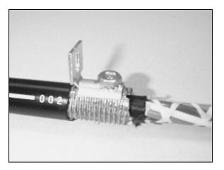
Figure 11 - Install top half of bond clamp.
