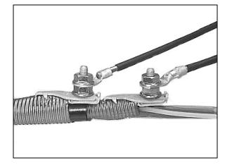
Figure 23 – Attach bond wires to the clamp studs.
