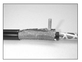
Figure 15 - Insert bottom half of bond clamp
