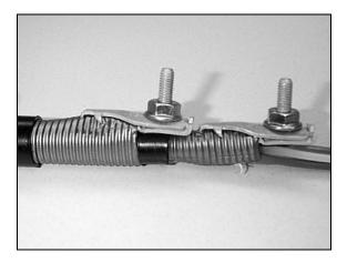
Figure 22 – Install Second Bond Clamp
