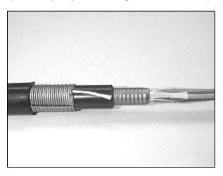
Figure 18 - Expose 1-inch of both armor layers.
