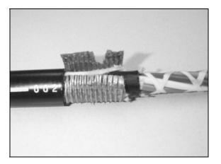
Figure 9 – Cut a slot in the armor.
