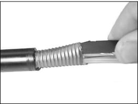
Figure 3 – Insert the plastic guard.
